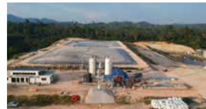
1.5MW FJP Biogas Plant with 2 Anaerobic Digesters
