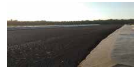
Covering of an Existing Anaerobic Pond for Samarahan Project
